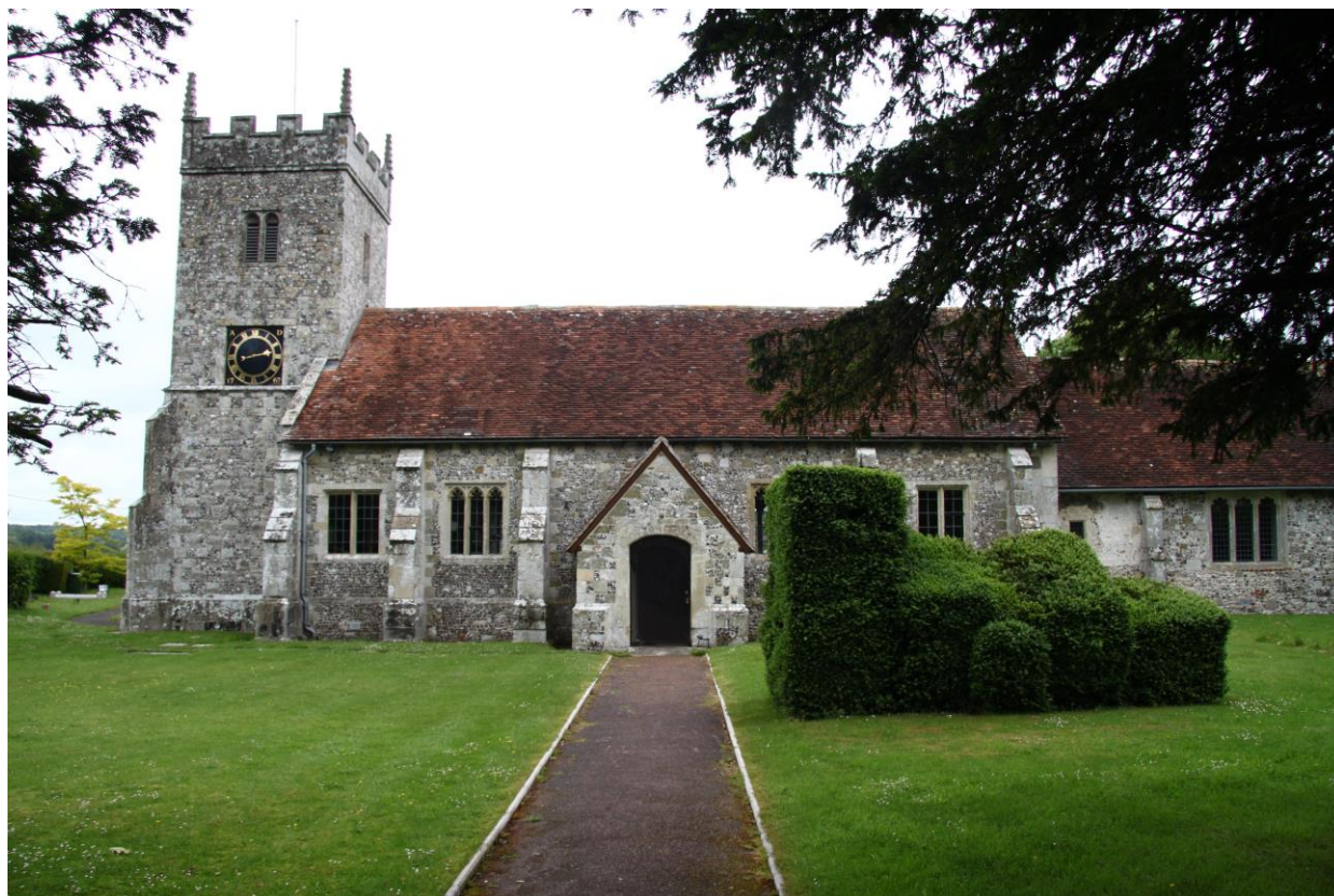
St. Lawrence Church, Stratford-sub-Castle
